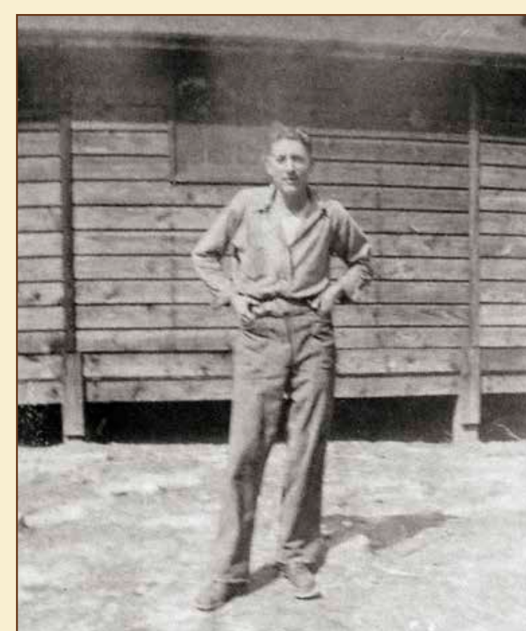
In this photo you can clearly see the modular sections that characterized CCC's portable buildings.
