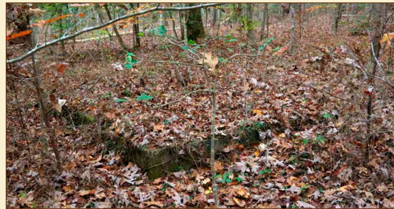
This foundation, as it appeared prior to being uncovered.
