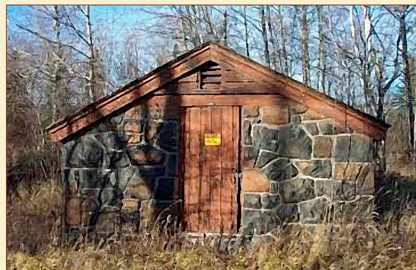
Though the ice house at Camp S-67 likely had wood siding rather than stone, the general shape and design of this CCC ice house, in Michigan, was likely quite similar.
